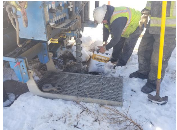
Photo #8 View of driller backfilling borehole 1358-13 (3) with bentonite chips.
