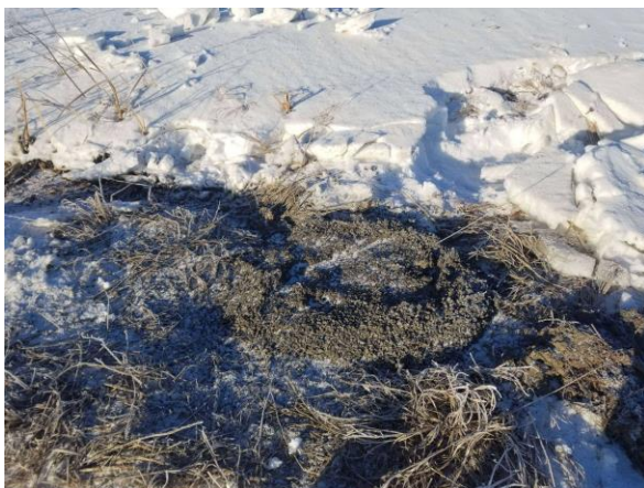
Photo #5 View of completed borehole 1358-13 (1).
