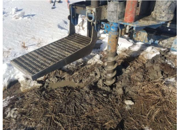
Photo #2 View at borehole 1358-13 (2) - groundwater stopped flowing at approximately 24 feet bgs.
