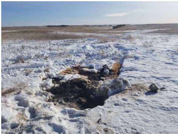
Photo #9 View south of completed borehole 1358-13 (3).
